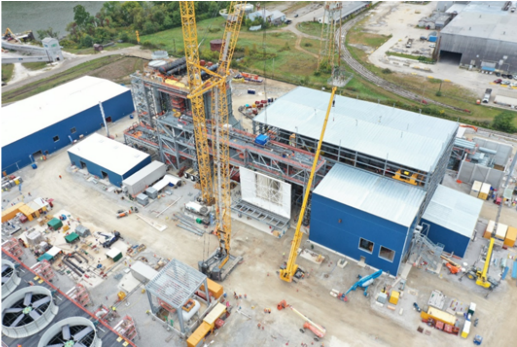
Long Ridge power plant under construction in Hannibal, Ohio. Photo courtesy of Kiewit.
