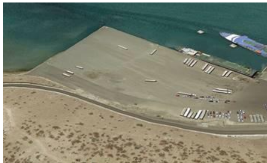
Q1 2019 Site fencing erected
