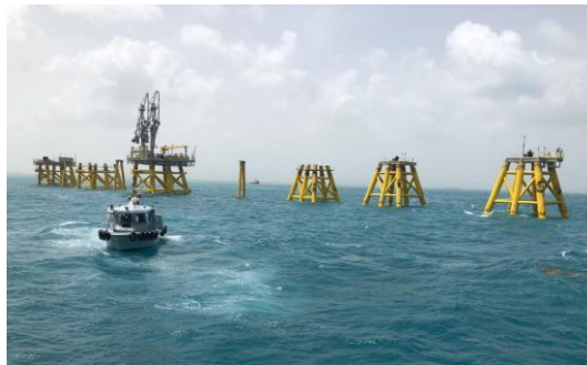
Q2 2018 Berthing dolphins under construction
