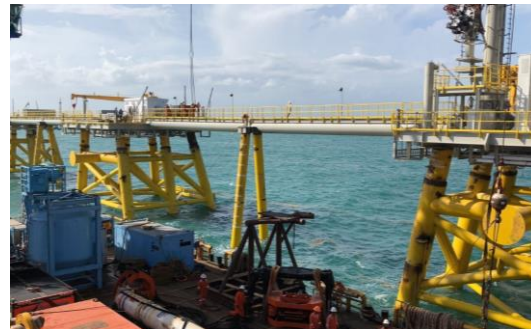
Q3 2018 Walkway and control center completed
