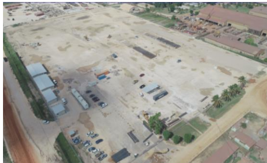
Q4 2018 Project site cleared
