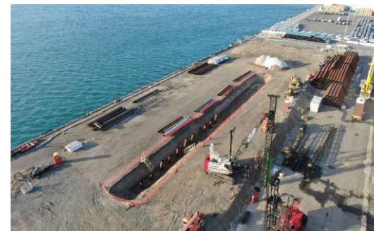
Q2 2019 Commencing berth repair (piling)
