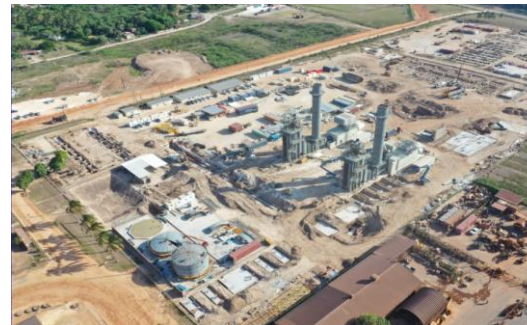
Q2 2019 ADO tanks & switchyard under construction
