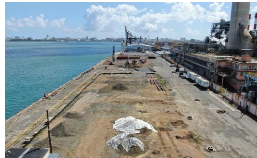
Q2 2019 Site cleared and ready for civil work
