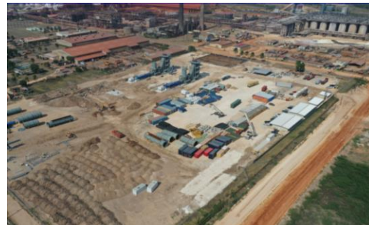
Q1 2019 Power island under construction
