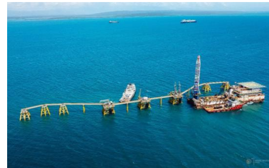
Q4 2018 Final offshore platform construction
